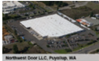
Northwest Door LLC, Puyallup, WA
